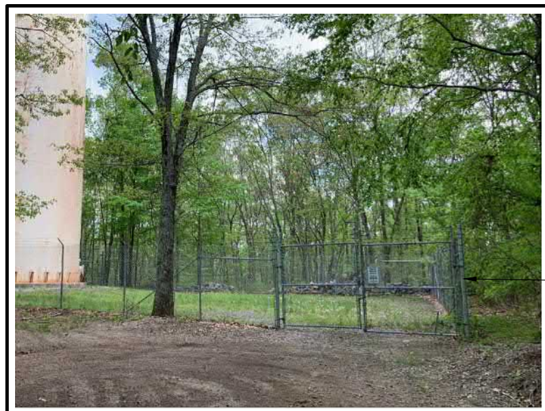
PHOTO 1 NEW TANK LOCATION
