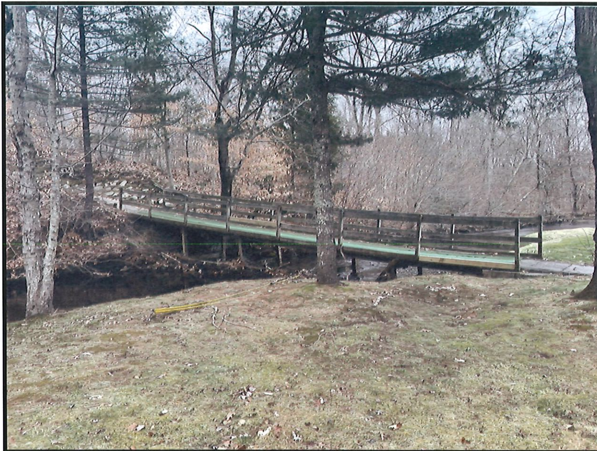
Picture 1: Existing cart/pedestrian bridge looking at upstream side (looking southeast)
