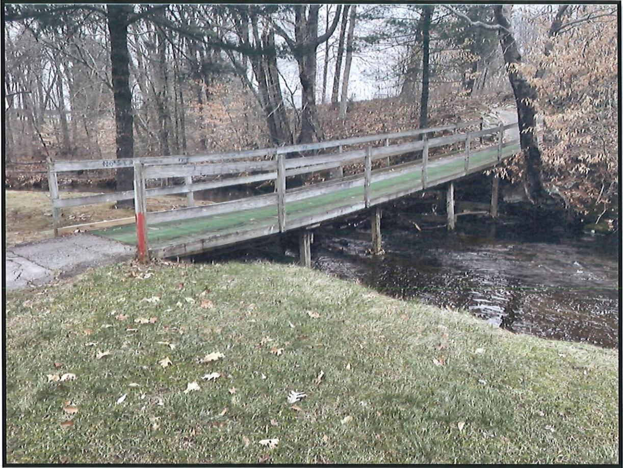
Picture 2: Existing cart/pedestrian bridge looking at downstream side (looking northeast)
