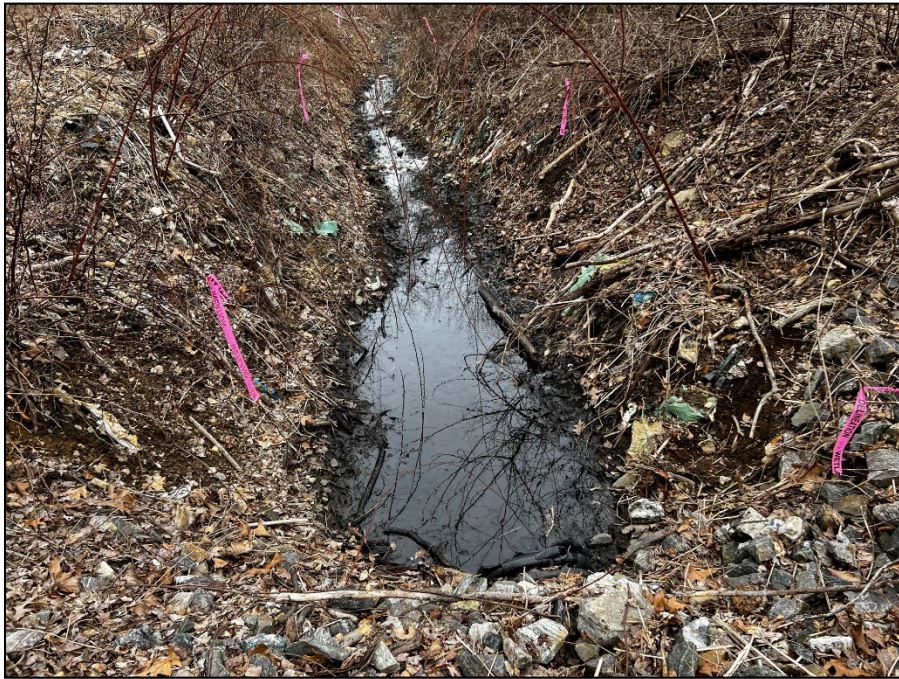
Photo 4: View of drainage ditch wetland near Oakdale Road.
