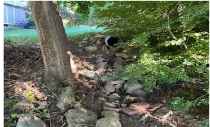
Culvert from Catch bason from Cedar Lane
