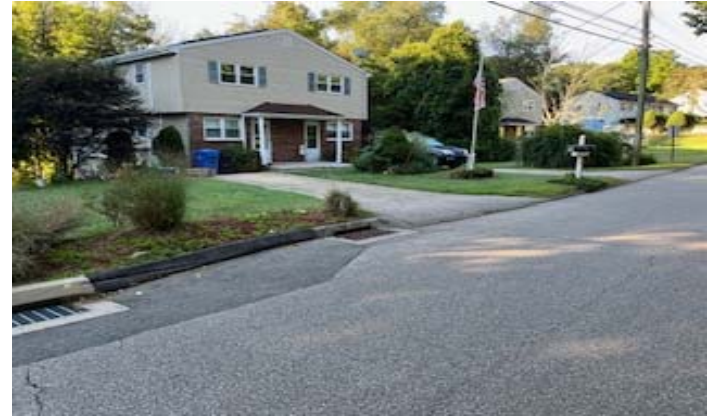
Catch basins on Cedar lane
