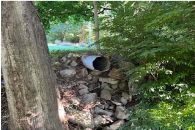
Culvert from Catch bason from Cedar Lane
