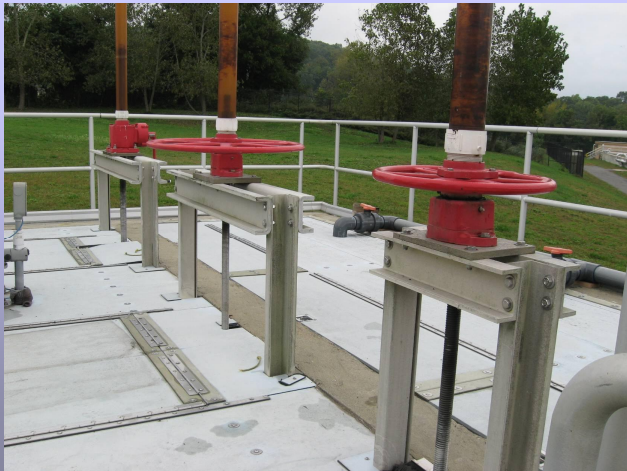
Flow distribution chamber
